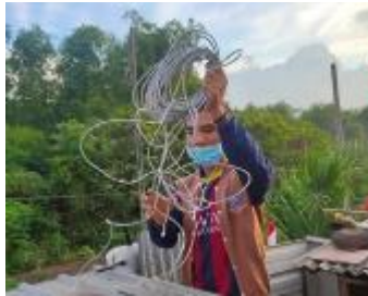
Gambar 2.9. Pemasangan Hospot Wifi
